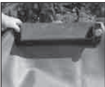
Fig. 32 Make sure you have a few inches of slack liner along the front base of your biofilter box
