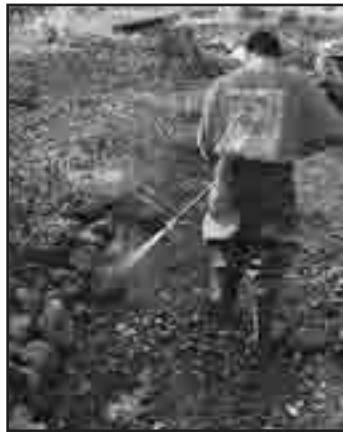
Fig. 52 Wash down the basin rocks to removed matted algae. Start at the top and work your way down, while pumping out the dirty water that is collecting on the bottom. Make sure not to scrub out all the algae; some will prove beneficial in developing your ecosystem.
