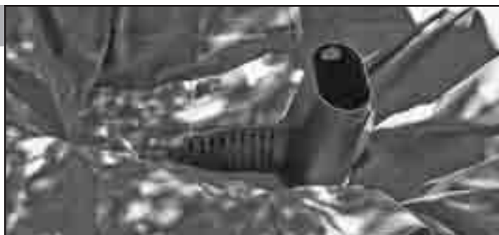
Fig. 17 Place The MicroSnorkel™ Vault and MicroCentipede™ Module on top of the liner.
