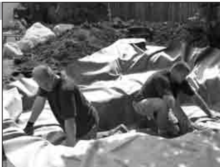
Fig. 16 Place the liner on top of the underlayment, following the same installation procedures. Make sure liner is positioned in such a way that allows it to extend and completely cover the opening on the MicroFalls®.
