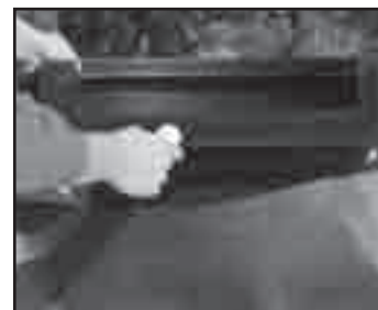
Fig. 35 Place a thick bead of silicone across the insert nuts.
