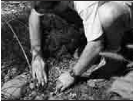
Fig. 45 Check the perimeter of the basin for any areas that are wet.
