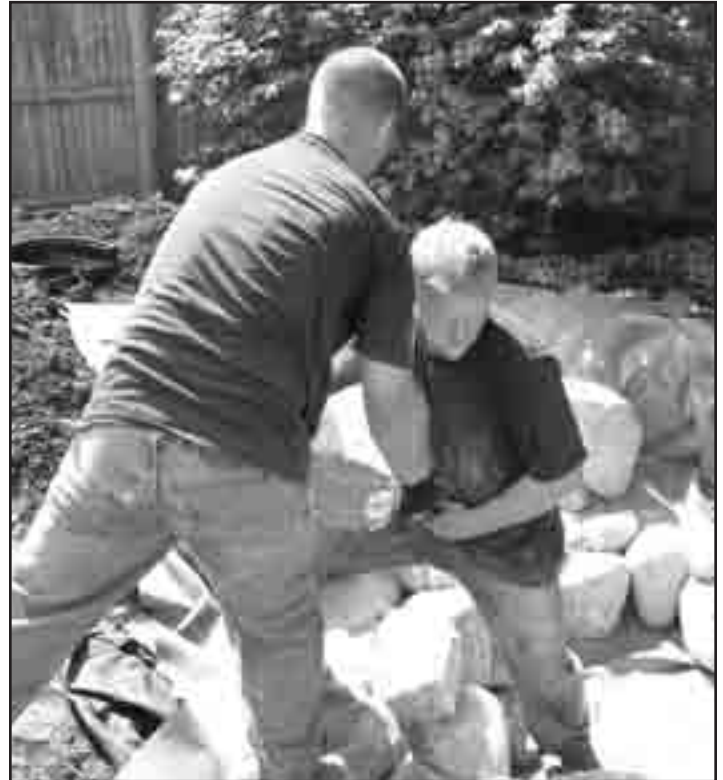
Fig. 27 Starting at the bottom set the largest character boulders first then fill in with the smaller ones.
