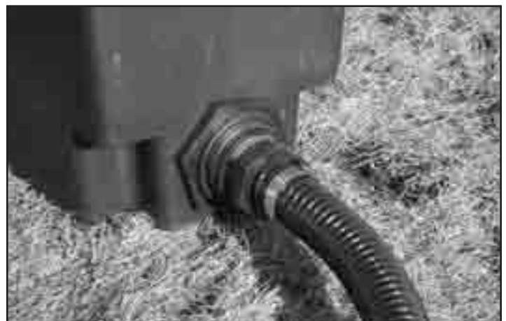
Fig. 7 Finished bulkhead assembly.
