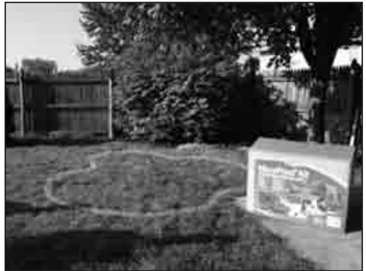
Fig. 1 Use a highly visible spray paint and outline the shape on the grass.
