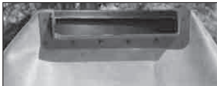
Fig. 38 Install the rest of the screws and remove extra liner, using the waterfall lip as a guide.
