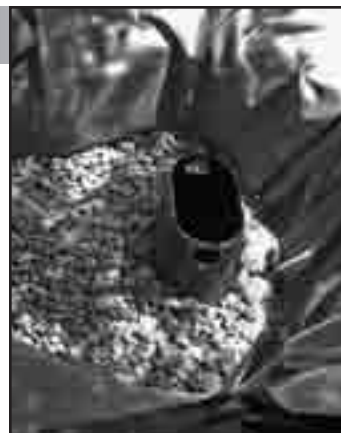
Fig. 25 Add gravel into the basin.
