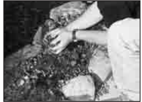
Fig. 47 Hide the exposed liner with gravel and mulch.
