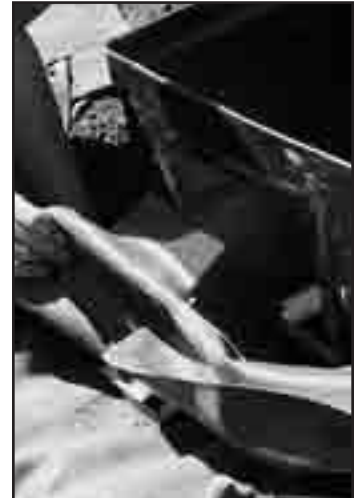
Fig. 24 Carefully replace the skimmer faceplate into the silicone lined opening.
