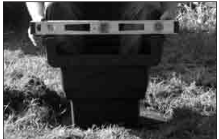
Fig. 6 Level the MicroFalls® side to side as well as front to back.
