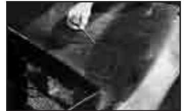
Fig. 19 Mark the skimmer opening on liner and cut an area 1.5" inside that mark.
